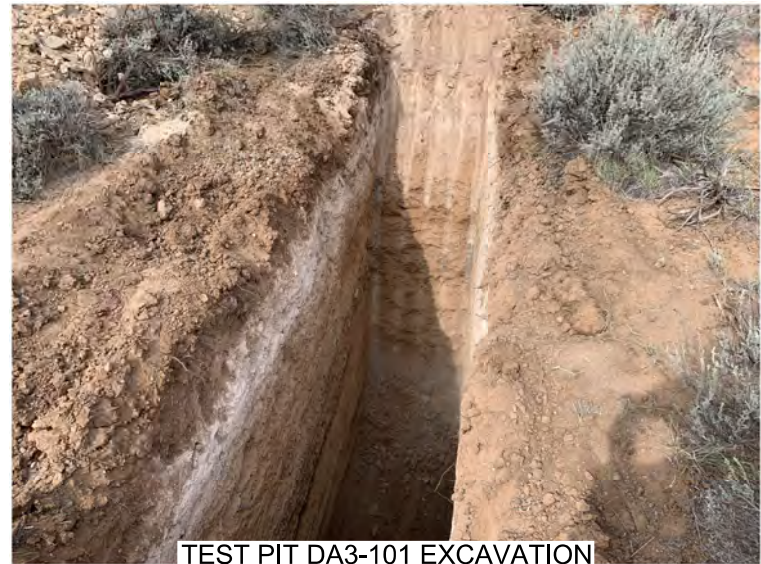
TEST PIT DA3-101 EXCAVATION
