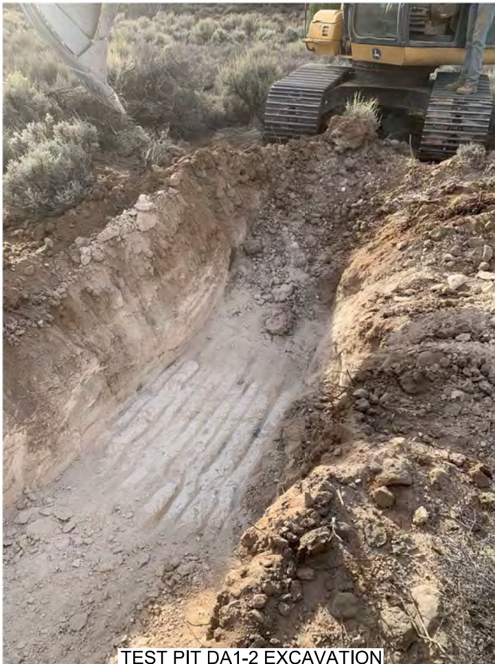
TEST PIT DA1-2 EXCAVATION
