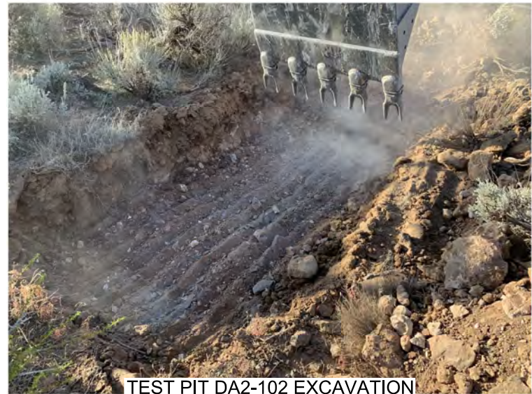
TEST PIT DA2-102 EXCAVATION
