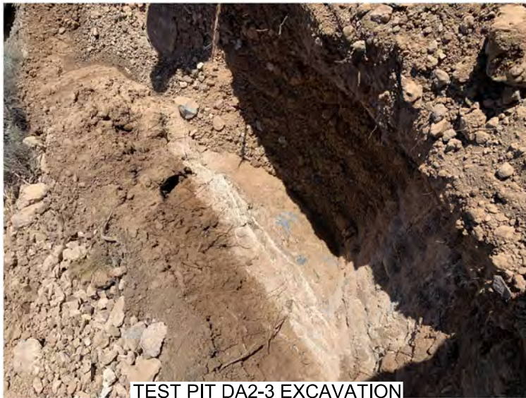
TEST PIT DA2-3 EXCAVATION
