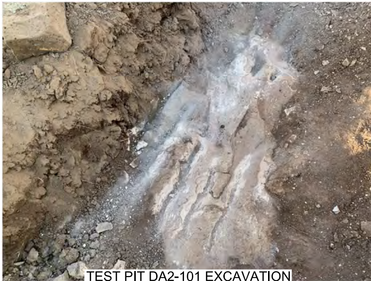
TEST PIT DA2-101 EXCAVATION
