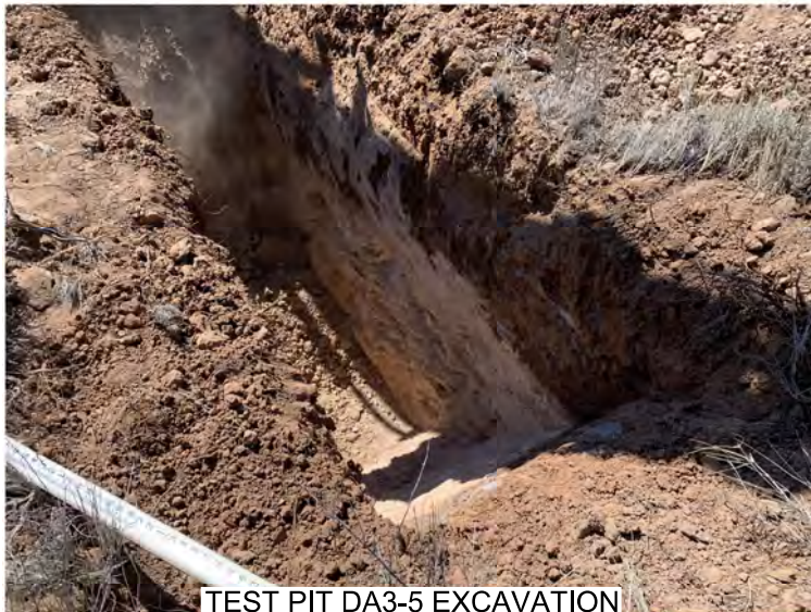
TEST PIT DA3-5 EXCAVATION
