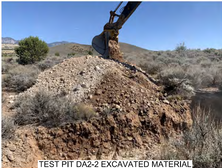
TEST PIT DA2-2 EXCAVATION
