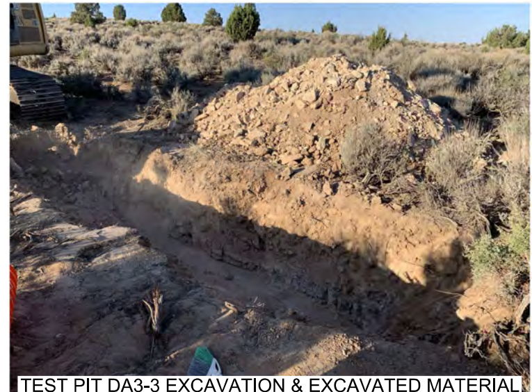
TEST PIT DA3-3 EXCAVATION & EXCAVATED MATERIAL
