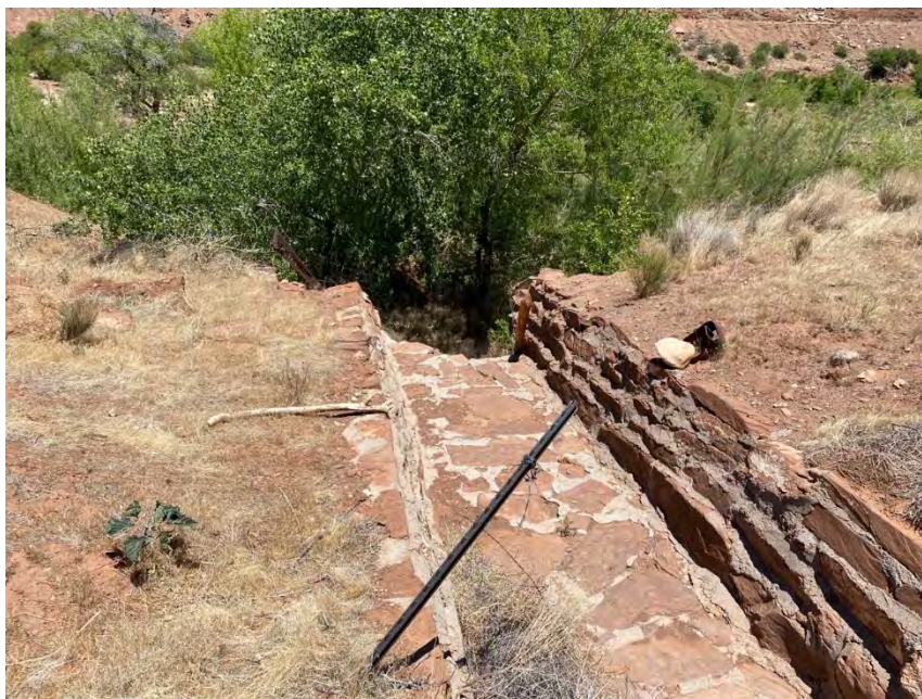
View of the improved section of Ditch 2 looking downstream where flows drop off the heavily eroded bank (facing northeast)
