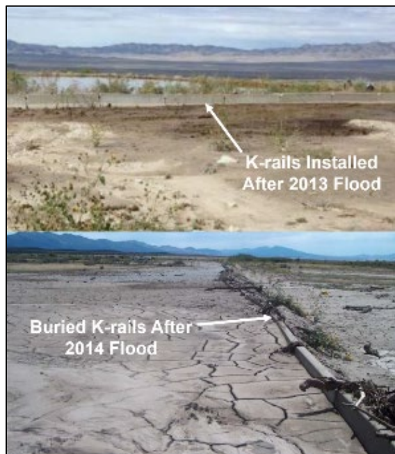
Figure 2-1. K-Rails 2013 and 2014 Flood
