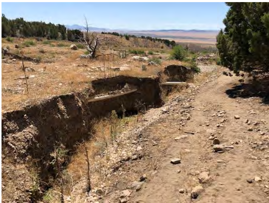
Figure 23. Destroyed Pipeline Example 1
