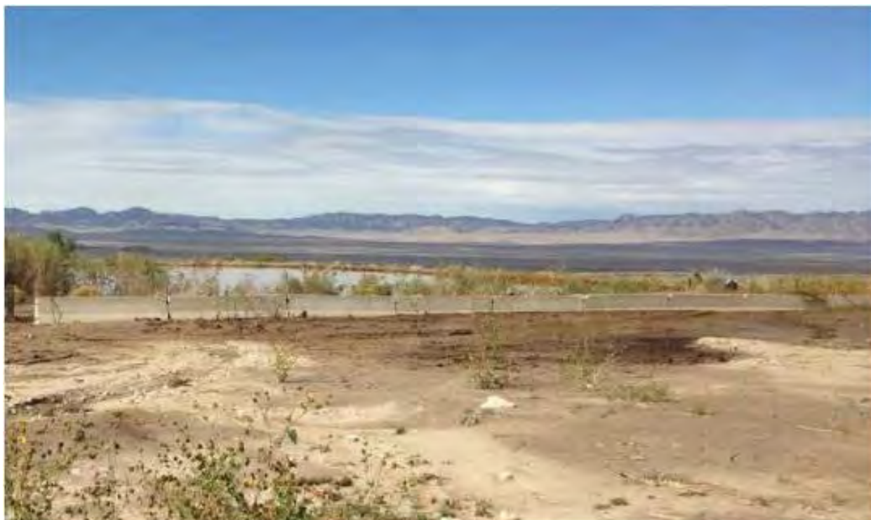
Figure 7. K-rails installed after 2013 flood event.
