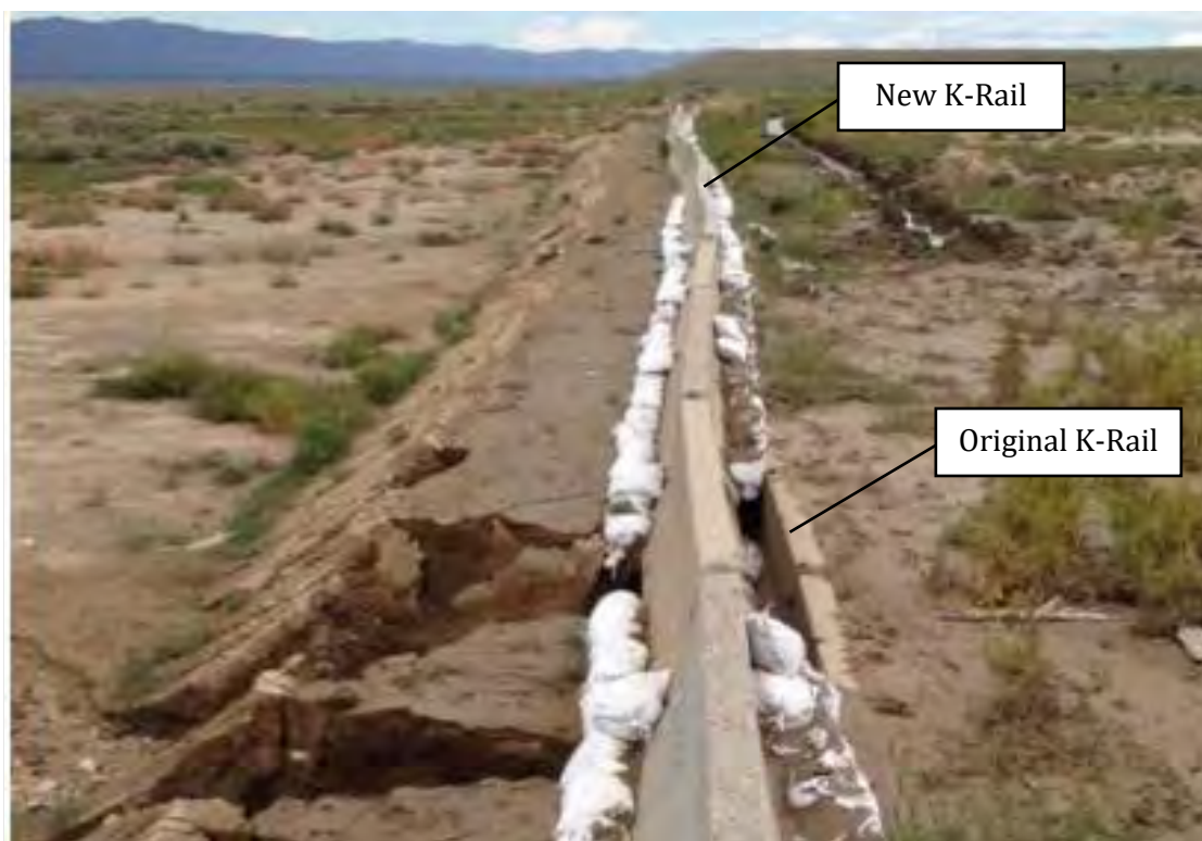
Figure 10. New K-rail installation after 2014 flood
