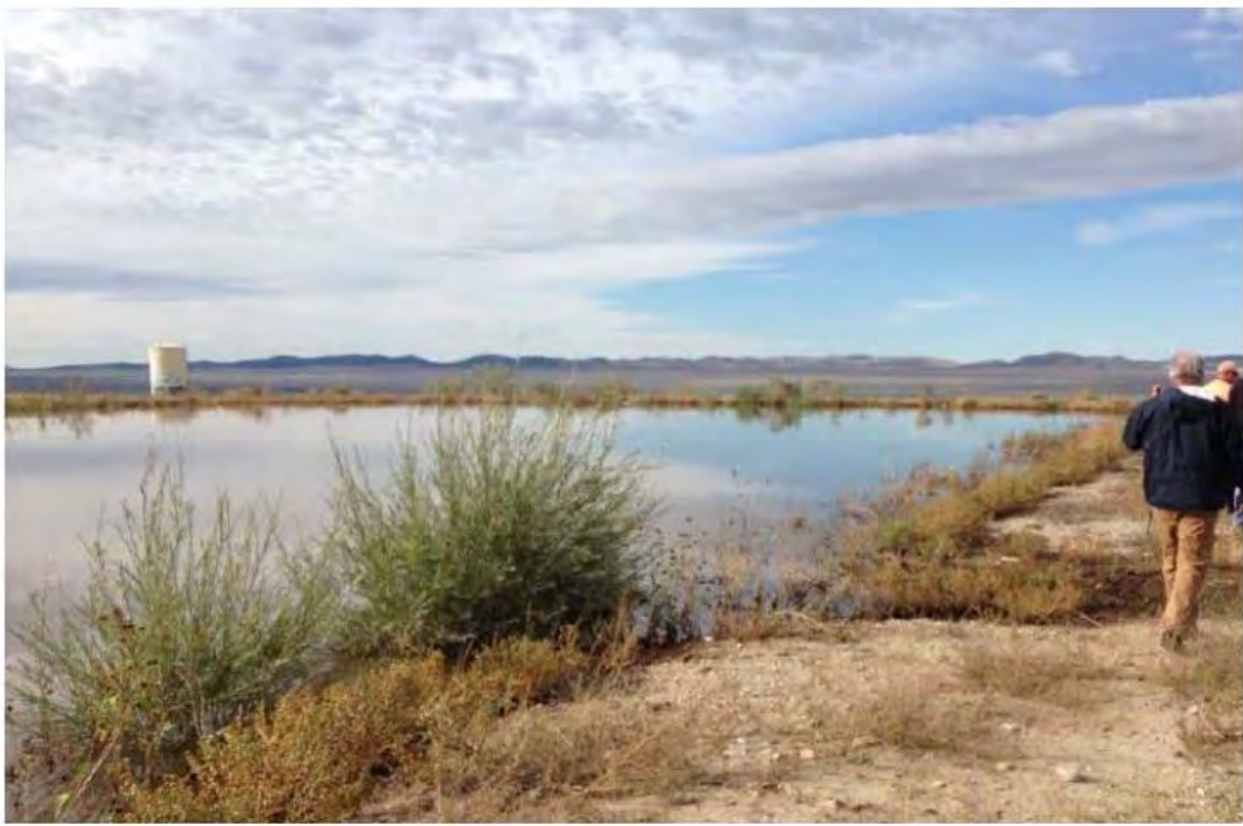
Figure 22. Irrigation Pond after Pond Outlet was Plugged by Flood Runoff in 2014
