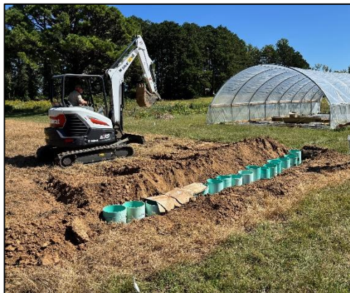
FIGURE 1. ERIN TAPLEY DIGS TRENCH FOR ROOT GROWTH CHAMBERS.
