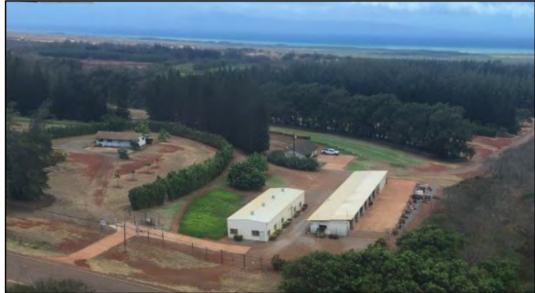
Figure 1. The Hoolehua Plant Materials Center occupies 80 acres in the central part of the island of Molokai, Hawaii.
