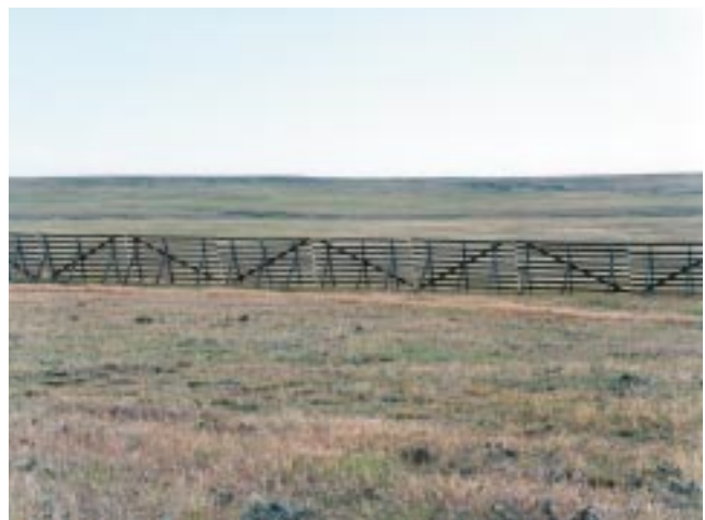
Figure 15. Where soils are too shallow, structured barriers are used to trap snow.
