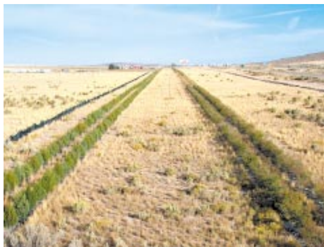
Figure 24. Double twin-row living snow fence installed along I-84 in southern Idaho.
