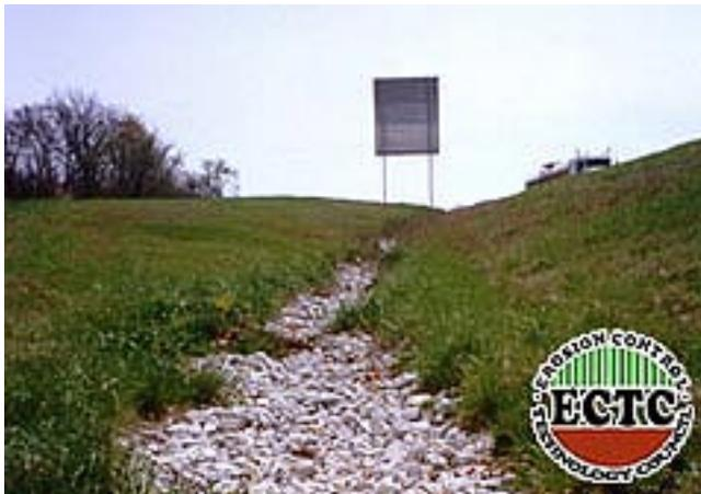
*Rip Rap rock used for erosion control in a water channel. Photo courtesy of the Erosion Control Technology Council.*
