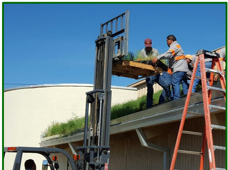
Green roof tray installation, photo TAMUK
