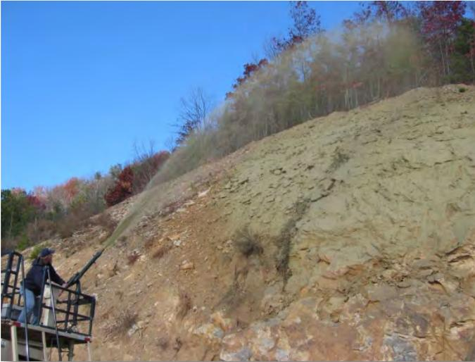
Figure 8. Seed mixture being hydro seeded onto the Foot Hills
