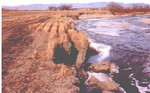
Cropland eroding into a stream. This field could have been protected with a properly managed riparian buffer. Photo by Rob Sampson, NRCS.
