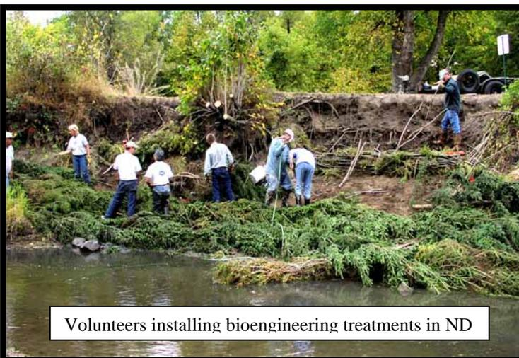
Streambank soil bioengineering projects are often very cost effective if applied appropriately. Erosion areas often begin small and eventually expand to a size requiring costly traditional engineering solutions. Installation of streambank soil bioengineered systems when the problem is small provides economic savings and minimizes potential construction impacts to adjoining resources. Many soil bioengineering projects can be installed by landowners and/or volunteers. The use of
