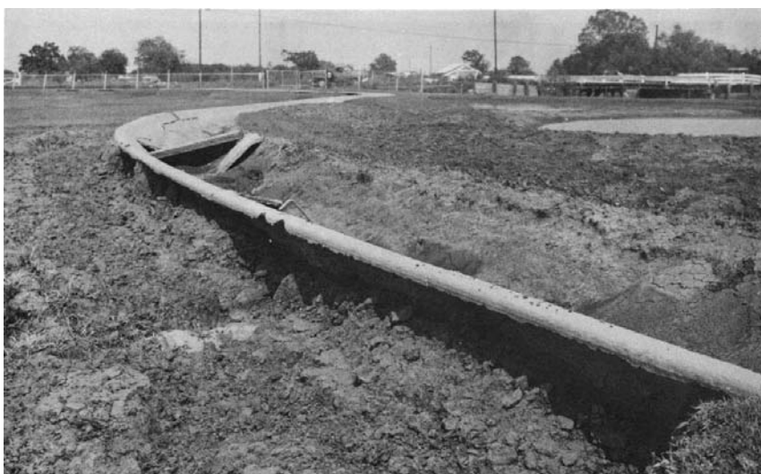
Figure 14.—A concrete-lined irrigation ditch on an area of Mangum soil has been severely damaged by floodwater.
