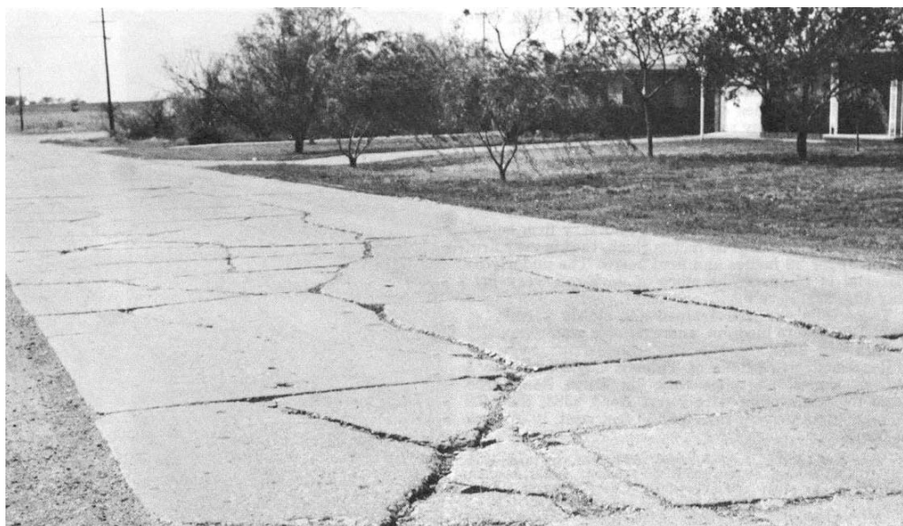
Figure 23.—Shrinking and swelling of this Tillman clay loam have severely cracked and damaged concrete street.
