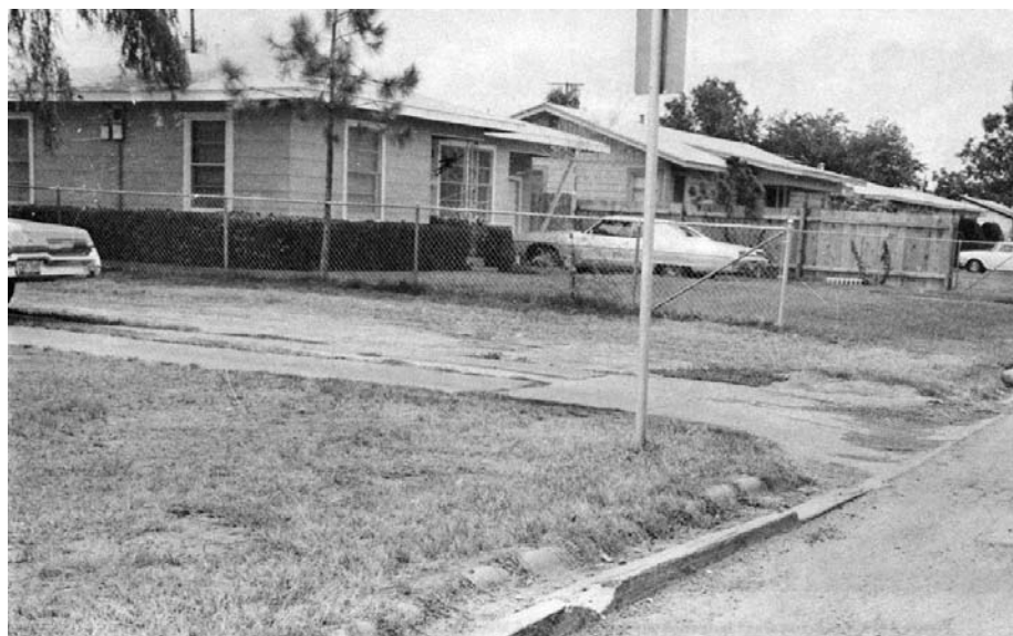
Figure 15.—Shrinking and swelling in an area of Mangum clay caused curb and street to crack and shift.
