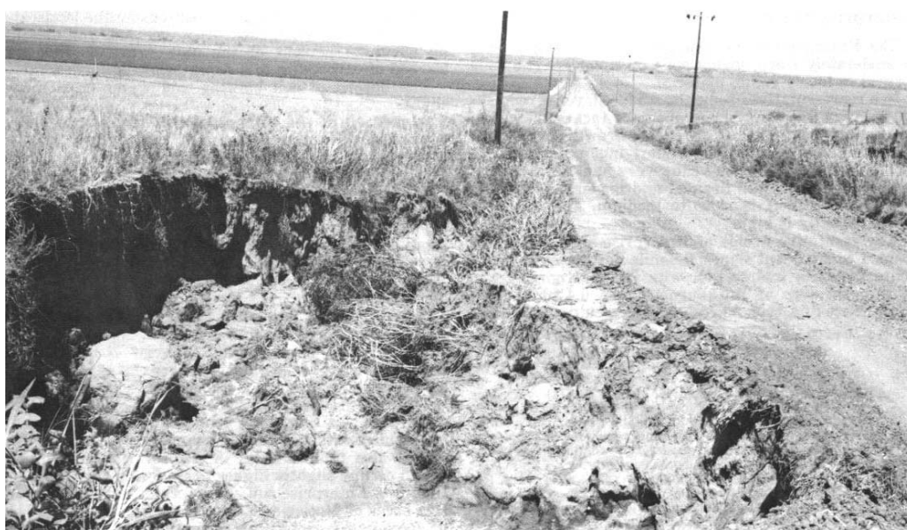
Figure 6.—Roadbank erosion on an area of Enterprise very fine sandy loam, 3 to 5 percent slopes.
