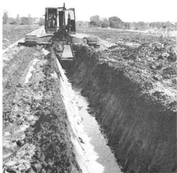
Figure 2.—Digging an open drainage ditch in Yonges loamy fine sand. (Capability unit IIw-3)
