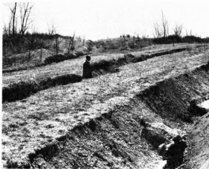
Figure 5.—This old roadway through an area of the Aura and Croom gravelly loams, 20 to 50 percent slopes, has been abandoned because erosion has been severe.
