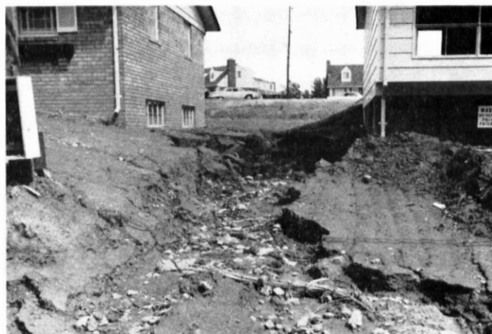
Figure 8. — Top: This land has been stripped of vegetation prior to building homes. No attempt has been made to control soil erosion, and every rain washes away some soil. Middle: Some houses have been built but still no attempt has been made to control erosion. The gullies and other soil erosion and the ruined drainage ditch at the left are the result. Bottom: When erosion is not controlled in residential areas, gullies may undermine the foundations as shown.
