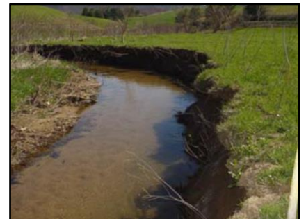
Before photo shows an eroded streambank.
