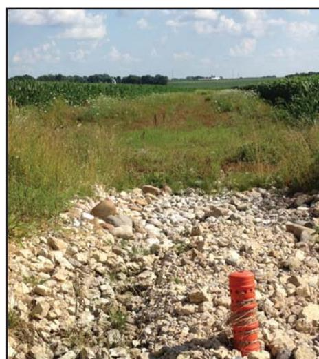
*Structural practices such as this grassed waterway and underground outlet capture the runoff from the surrounding fields, preventing erosion and improving water quality.*
