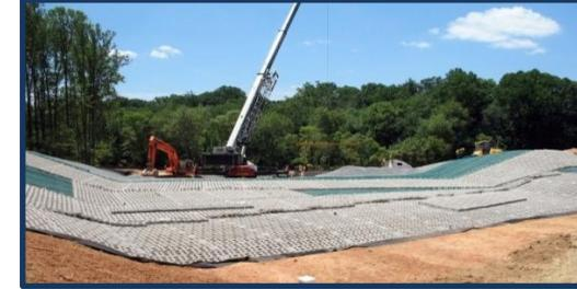
Articulated concrete blocks were placed in the auxiliary spillway.
