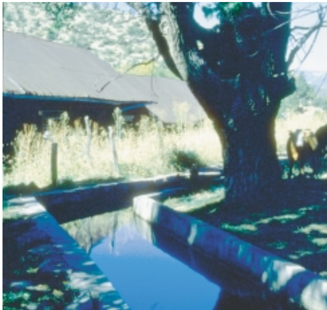
Fig. I.2: Concrete-lined channel. Stream systems across the nation have been altered for a wide variety of purposes.
