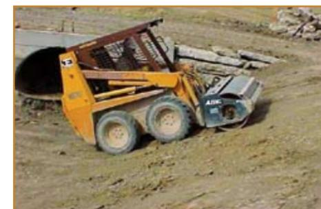
Construction grading compacts the soil and exposes land to erosive rain and wind.
