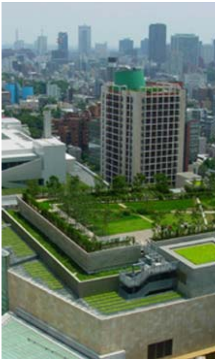
Example of green roofs.
