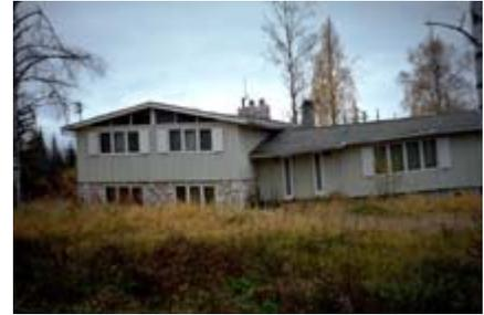
**Figure 5.—The result of building a conventional foundation on permafrost-affected soils containing massive ice. Heat transfer from the house resulted in melting of the ice and displacement of the foundation.**
