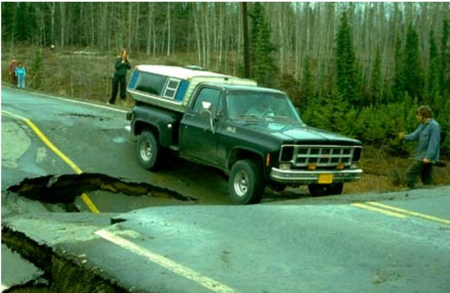
**Figure 4.—Collapse of a section of the Alaska Highway in 1982 resulting from melting of massive ice under the roadbed. (Photo by Joe Moore, USDA, NRCS.)**
