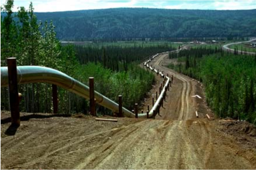
Figure 3.—Permafrost-affected soils with loamy textures become saturated and unstable if allowed to thaw. In areas that include these soils, the trans-Alaska oil pipeline is elevated above the ground.
