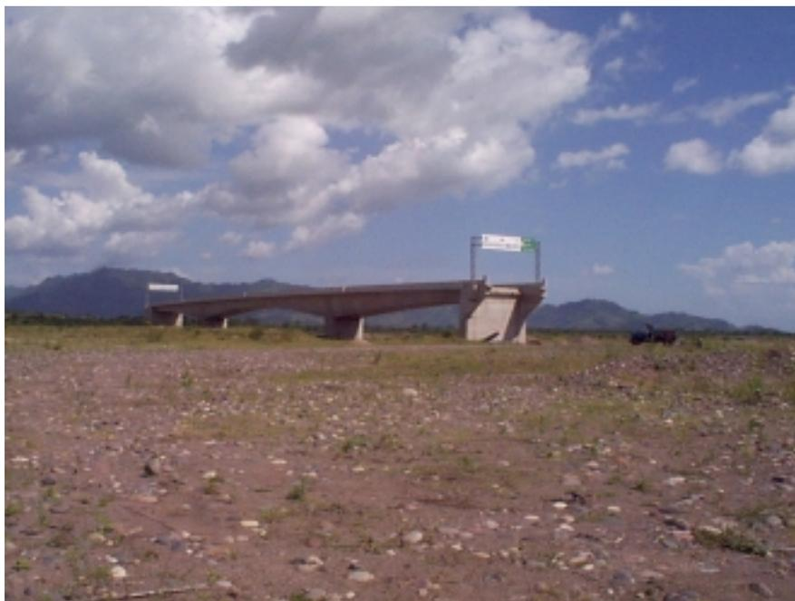
Figure 1.—A bridge that was in use for only 6 months before Hurricane Mitch swept part of it away.
