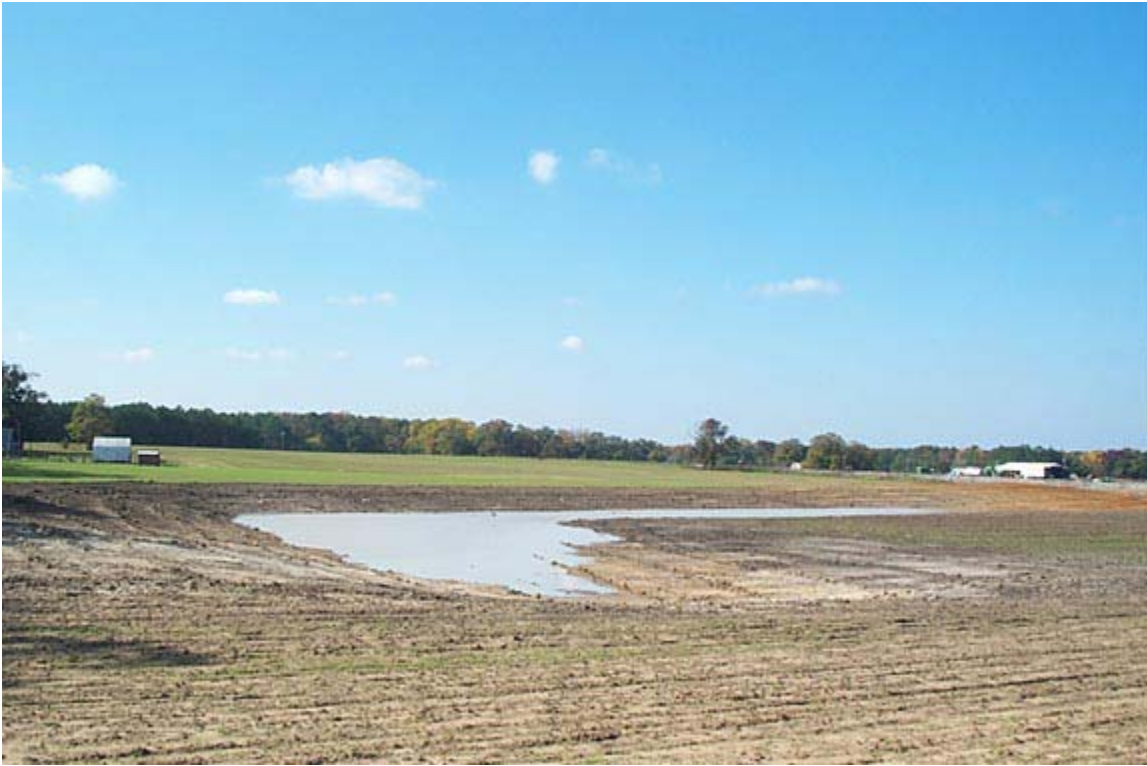
Swale and adjacent down slope ridge. Slopes of 20:1.
