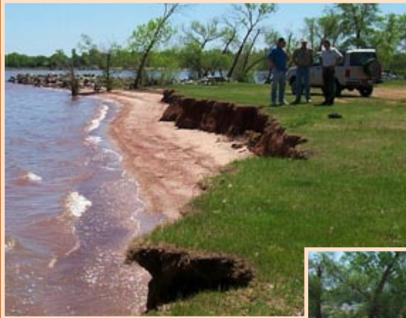
Shoreline erosion before (above) and six months after (right) bioengineering installation. Similar treatment is planned for select reaches of shoreline at Lake Carl Blackwell, near Stillwater, Oklahoma.
