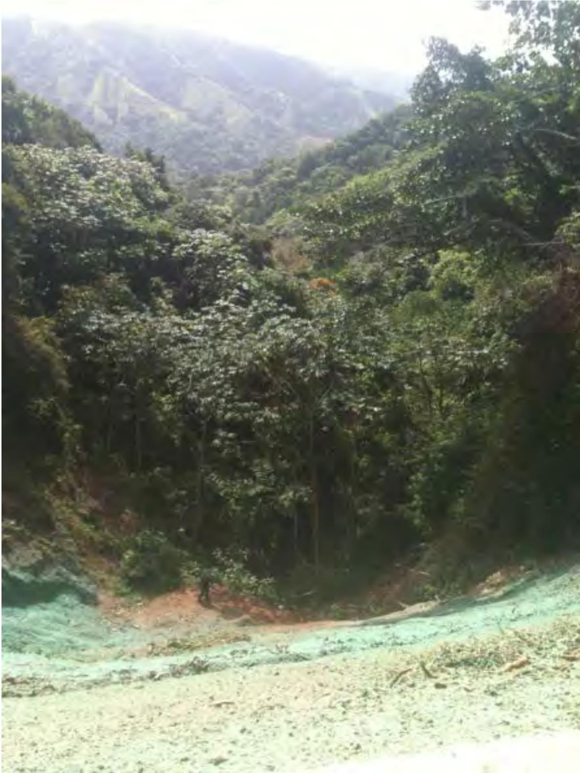
**Figure 4. Hydromulching complete on the 70% slope plots**
