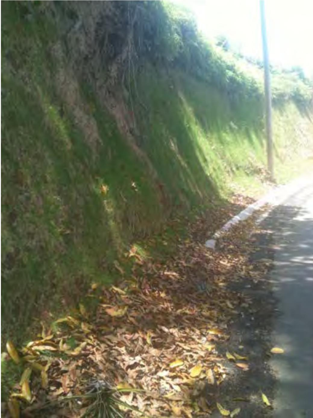
**Figure 9. Grass coverage on Plot #2 using Flexterra BFM**
