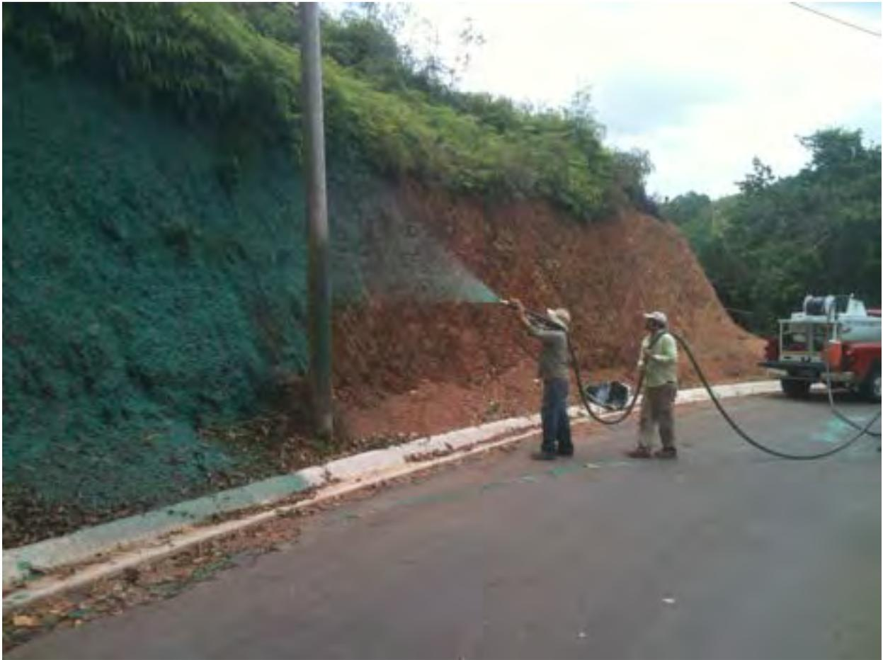
Figure 5. Applying hydromulch to the 85% slope in Plot #2
