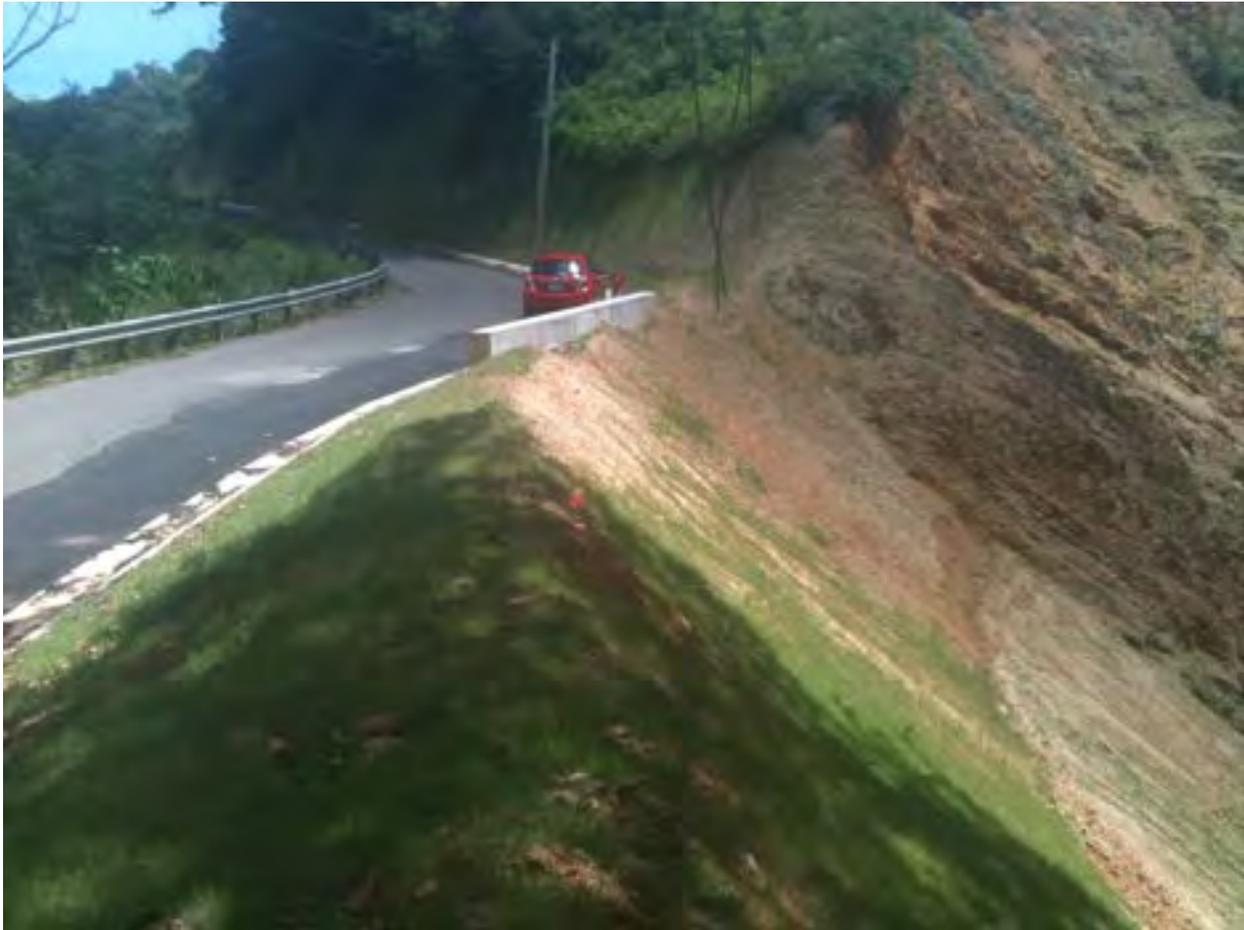
Figure 6. 7-23-12 Note Plot 3 with 50% vegetative cover and less vigorous grass growth was a thinner application of Flexterra (BFM) but also in an area with full sun and and high proportion of rock/consolidated material
