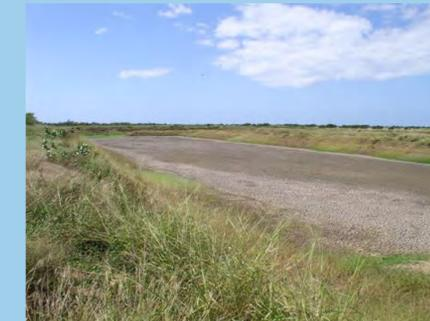
Basins will be built in Lower Río Loco to trap sediment to reduce siltation of nearshore reefs.
