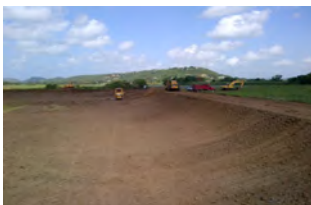
Irrigation Water Reservoir 3 under construction on Santa Rita Farm, Guanica, P.R.
