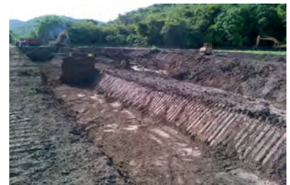
Sediment Basin B under construction at Santa Rita Farm, Guanica, P.R.
