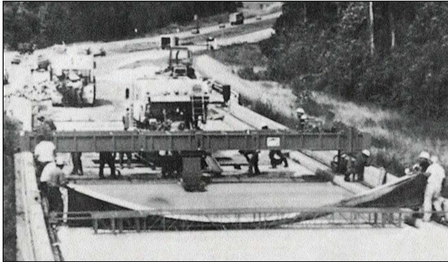
Figure 3. Continuous wet curing is recommended during hot weather. The curing cover used here is burlap with a polyethylene coating.
