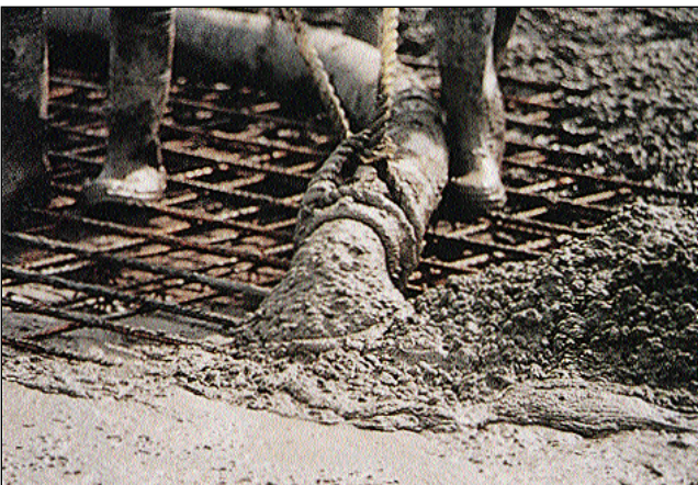
Superplasticized concrete pumps easily and arrives workable. For maximum effectiveness, however, superplasticizers must be added to the mix at the right time.
