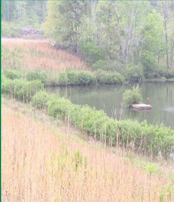
*Trees and shrubs need to be cut off the front slope and riser of this watershed dam.*
