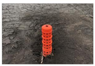
underground outlet can be installed when surface outlets are impractical because of stability problems, climatic conditions, land use, farmability, or equipment traffic. An underground outlet can be used as the only outlet for a structure or practice or it may be used in combination with other types of outlets.
