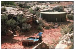
This practice involvestreating awatershed or portion of a watershed to increase, collect, and store runoff water. It may also involve installing curbs and/or diversions to direct the runoff water to a storage facility. The contributing area may be rock outcrops, paved areas, or other impervious areas that yield high rates of runoff. The contributing areamay requiretreatmentwith material such as asphalt, wax, rubber, plastic, concrete, metal, or other impervious material.
