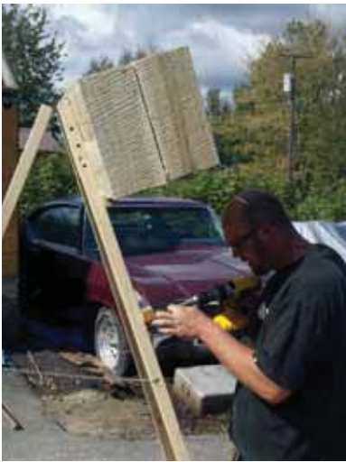
Maverick Deckert constructing new booths for The Alaska Farmland Trust.
