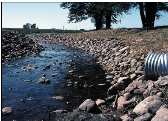
Figure 6. Rock rip-rap on a previously eroding streambank.
