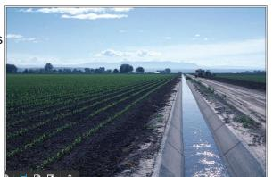
This practice applies to constructed ditches that are subject to erosion or excessive seepage and are integral parts of an irrigation water distribution or conveyance system.
