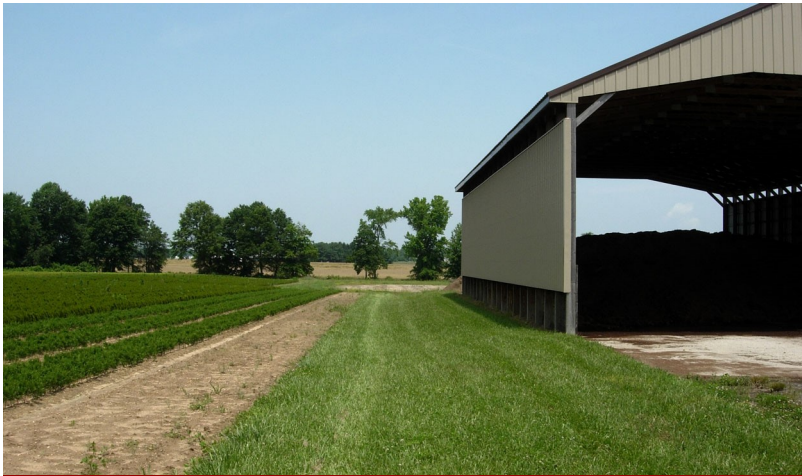
Grass filter strips surround structure to prevent excess runoff from seeping into the groundwater.
