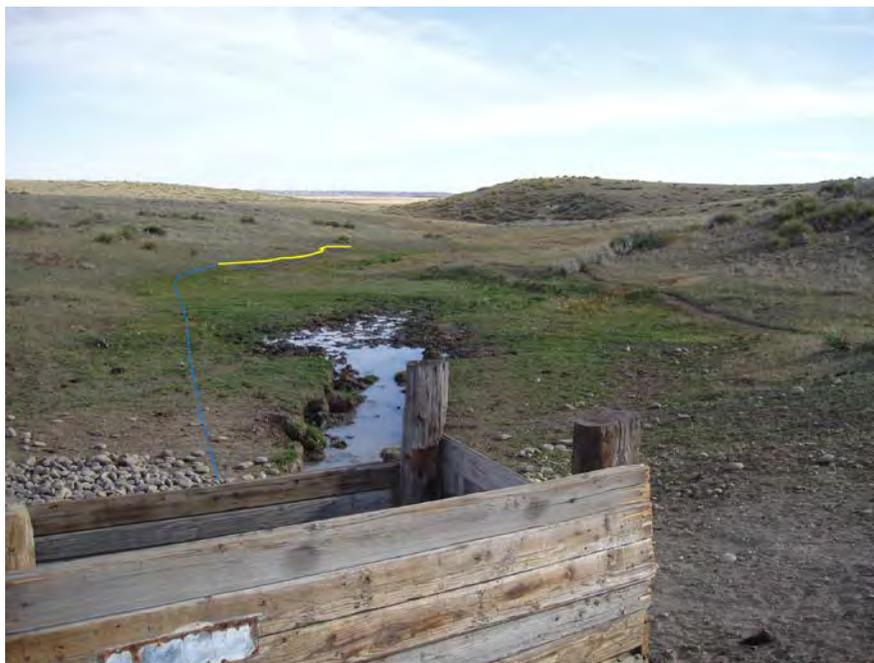
Figure 1. Re-create the seep by running the tank overflow to a similar slope position as occupied by the drained or partially drained seep above the tank – new seep created by perforated pipe shown in yellow. Fence off the seeps if necessary to prevent trampling
