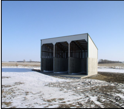
Static Pile, Concrete Bins
