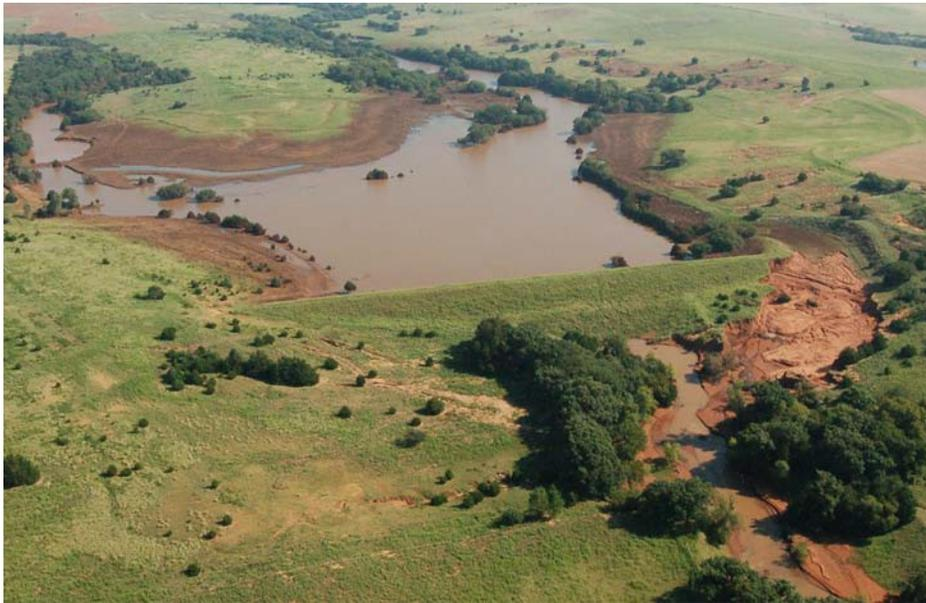
The auxiliary spillway of Sugar Creek Watershed Dam No. L-43 was damaged in August 2007, when the dam's watershed received 8.3+ inches of rain in a 6-hour period.
