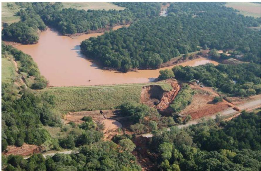
Damage to Sugar Creek Watershed Dam No. L-44 as a result of 8.3+ inches of rain in a 6-hour period in August 2007.
