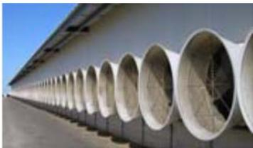
Exhaust fans are used to pull outside air through a building. They are typically used in tunnel or cross ventilation systems.
