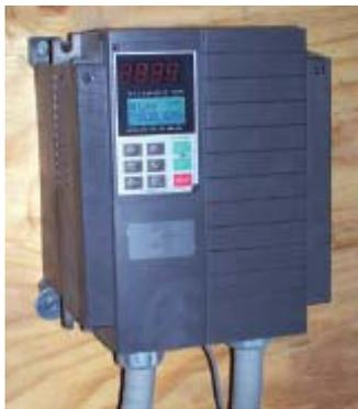
A variable speed drive varies the speed of an electric motor in order to more closely match demand and reduce energy consumption. They are especially useful on equipment that runs intermittently because they can reduce on/off cycling of the motor which reduces wear on the motor and can extend equipment life.
