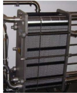
Well water precoolers are heat exchange units that use well water to cool milk before it reaches the bulk tank. The warmed water can be used for livestock watering or washing. Plate coolers can counteract benefits of a compressor heat recovery system because they reduce
