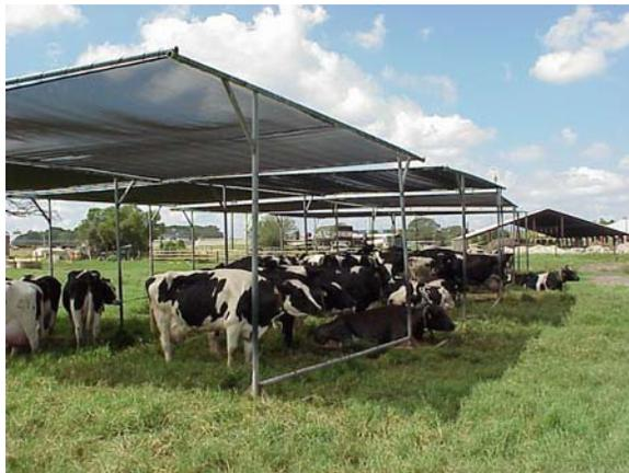
**Orientation.** Orient the longest axis in a north to south direction to maximize the amount of shade and to allow sunlight to dry the area under the structure.
