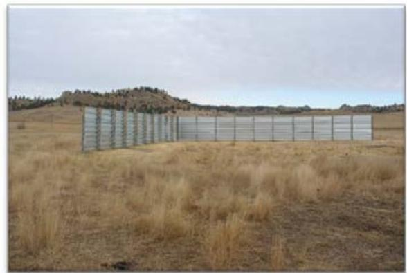
Locate the shelter on level, uninterrupted terrain, if possible. If the shelter must be located downwind of a hill, place the shelter as far downwind as possible. A shelter upwind of a hill shall be placed a minimum of 75 times the shelter height upwind of the base of the hill.
