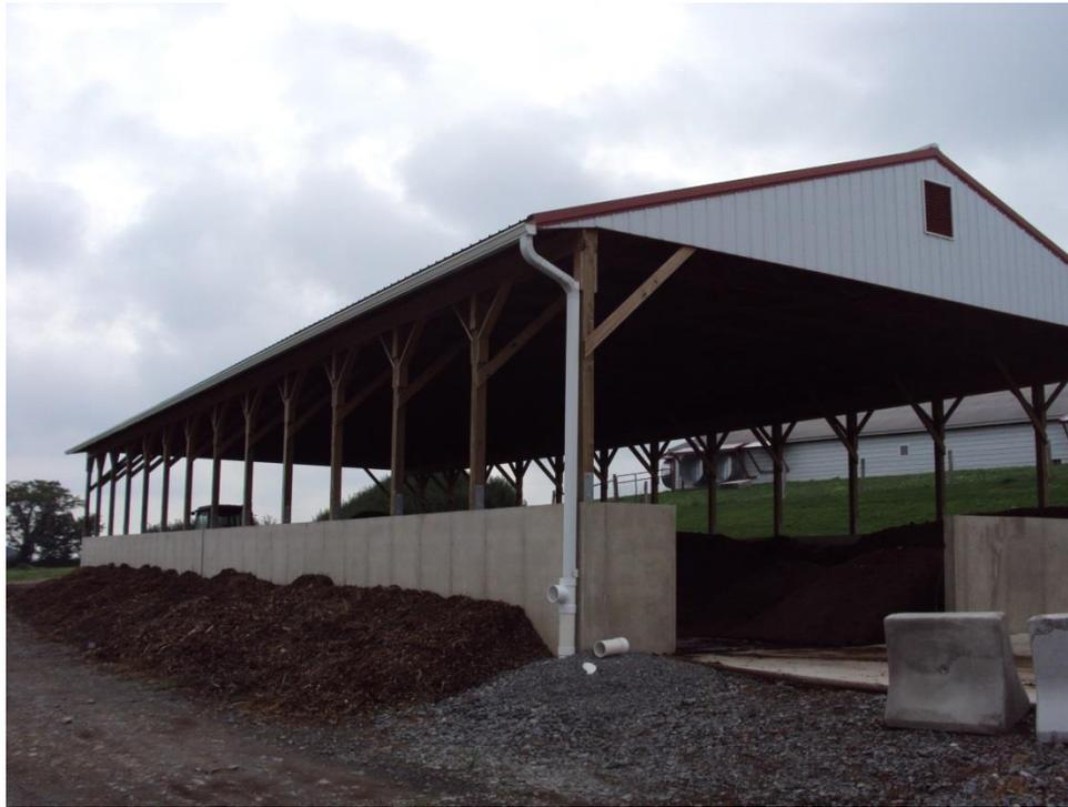
Dave Reifsneider's roofed stacking area. Note the overflow on the downspouts in case the infiltration trench "backs up".
