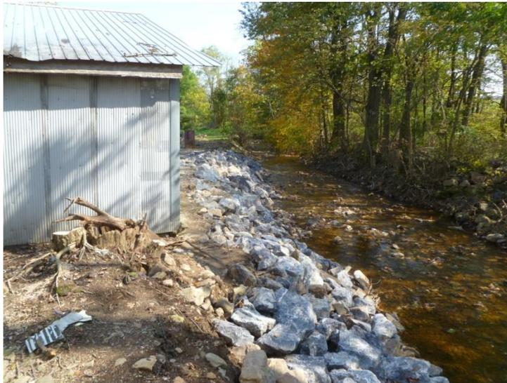
Dry Run, Center Township- After: Rip Rap secures the stream bank to protect it from erosion.
