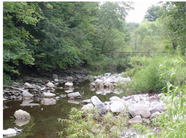
*To encourage trout to inhabit more areas of the West Branch Conneaut stream in Erie, PA, five stone deflectors with J hooks were installed to provide current breaks, deeper holding water, and habitat for insects (to provide food for trout).*
