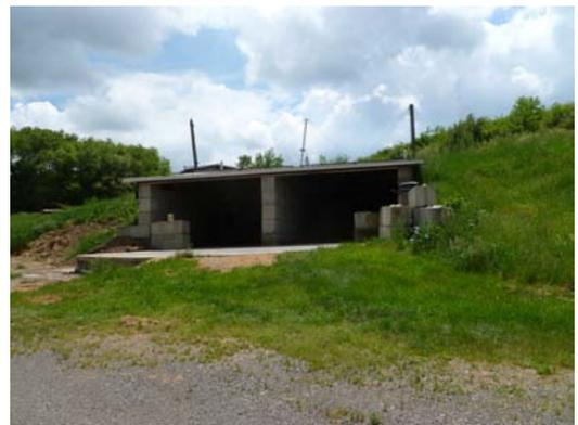
Fertilizer storage. Top rolls back for easy filling. Loads out from below.
