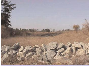
Rip Rap Used to slow water and filter sediment
