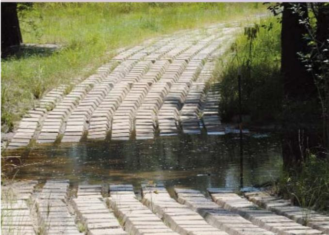
This is one of 12 stream crossings installed on the Edgy’s property by WRP funds. Stream crossings cut down on soil erosion and improve water quality
