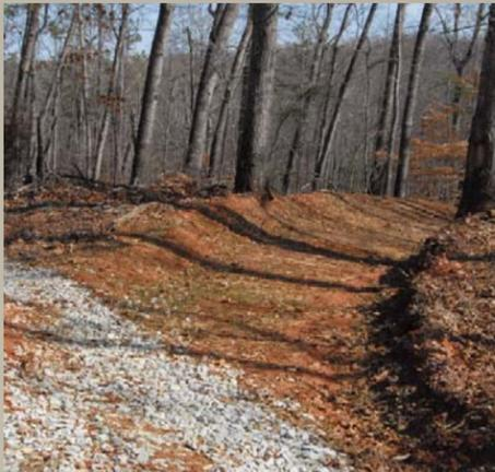
A broad base dip located at a critical point along the road moves the rain water off the road.
