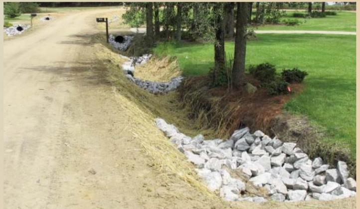
Dirt road prior to paving. Storm drain outlet protection and rock check dams were installed throughout the drainage system in order to reduce water velocities and trap sedimentation.
