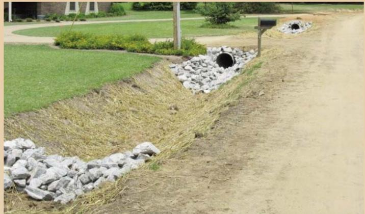
Drainage ditches that were filled with sedimentation were reclaimed. Temporary and permanent vegetation was planted and mulch was applied to disturbed areas.
